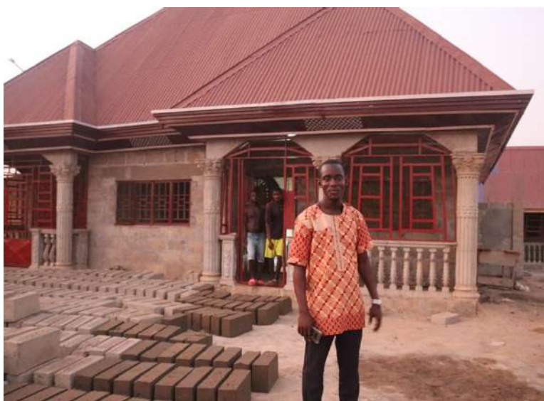
Abdulai at one of his construction sites
